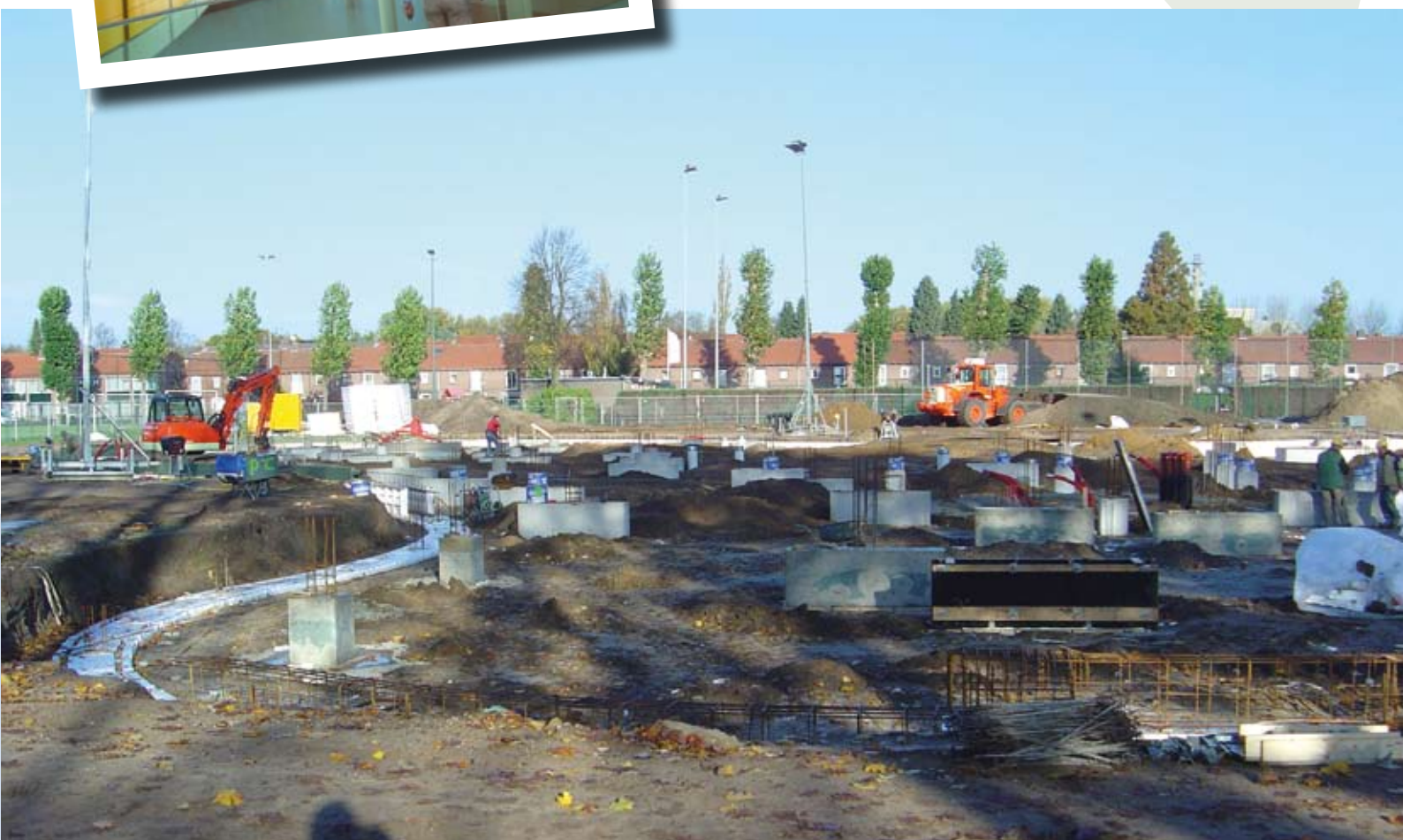
Groundwork in early November 2009, before construction of the school building commenced.
